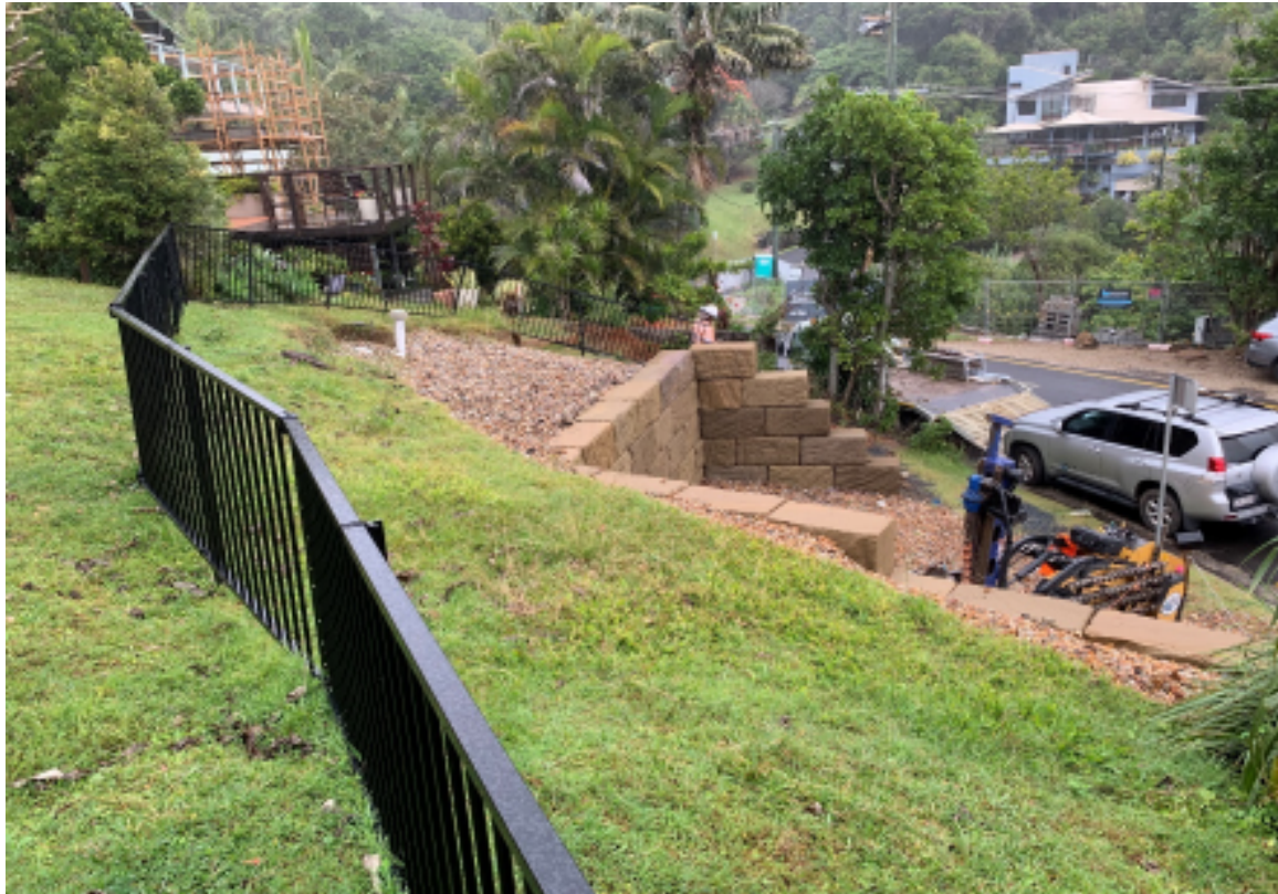
Plate 5 – Sandstone block retaining wall downslope of existing residence.
