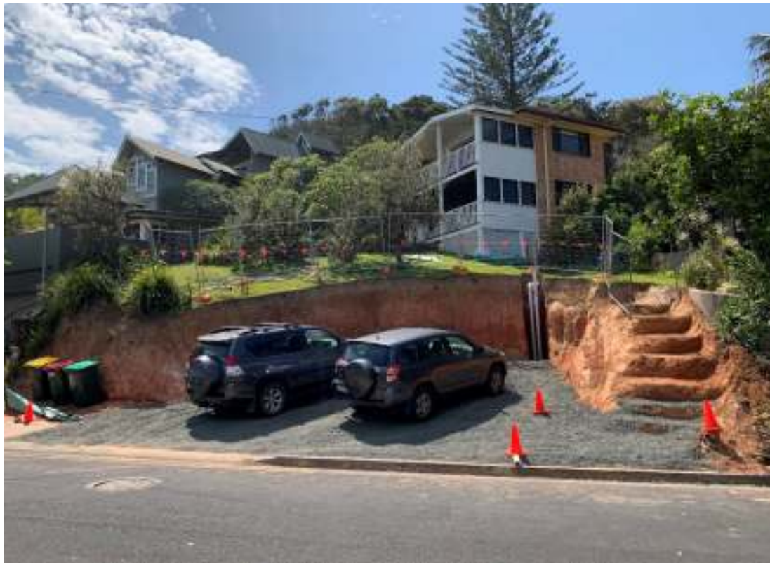
Plate 2 – Excavation prior to being retained by sandstone block retaining wall. Excavation exposes natural clay soil in upper section and weathered rock in the base.
